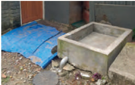
Black and Grey water pipes from households connected to common underground pipe leading to settling tank
