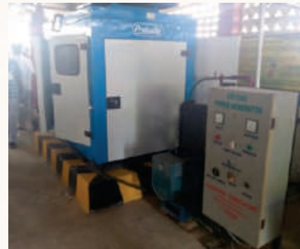
Biogas power generator
