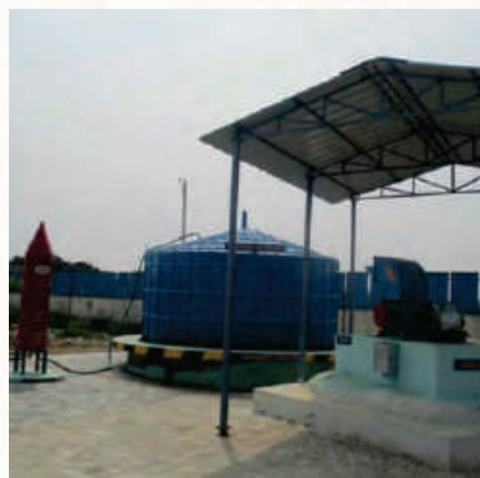
50 cubic meter Biomethanation Plant
