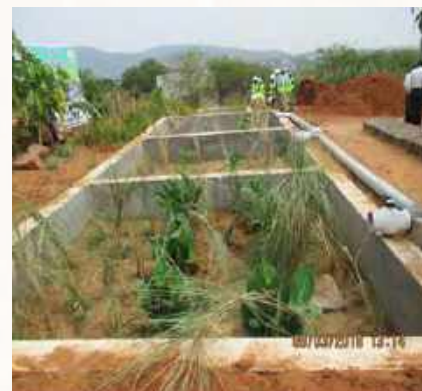
Septage from Feeding Tank is led into Vertical-flow Constructed Wetland
