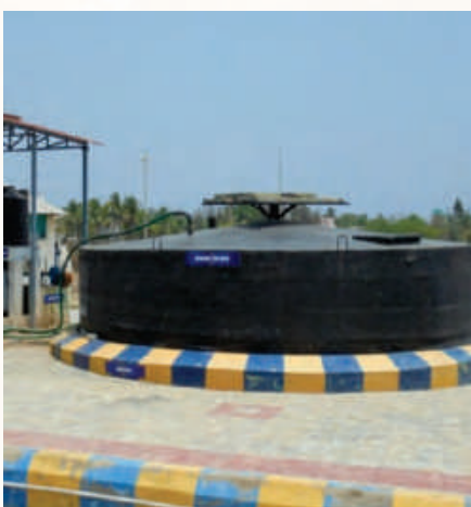
50 cubic meter Biomethanation Plant
