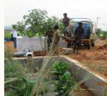
Septage from Feeding Tank is led into Vertical-flow Constructed Wetland
