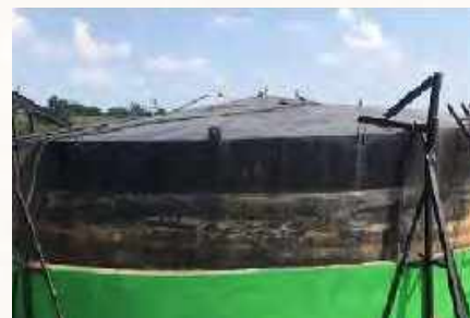
Floating dome Digester
