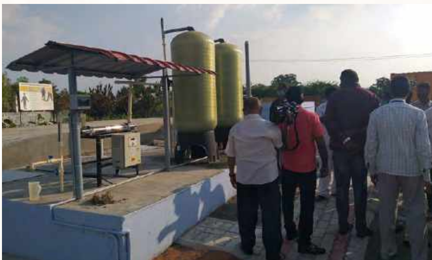
Pressure Sand Filter (PSF), Activated Carbon Filter (ACF) and UV Disinfection Unit
