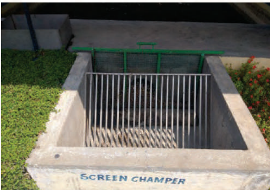
Screened Inlet Chamber
