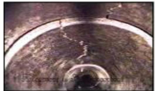
Photographs showing Structural Damage and Longitudinal cracked condition of the Sewer
