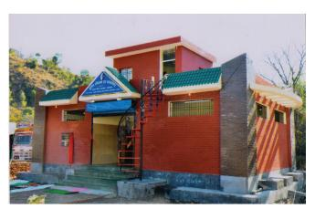
An example of: PT constructed using Cement blocks available locally
