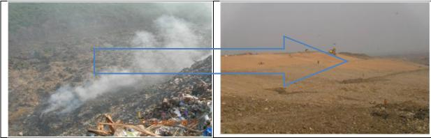
Pictures showing land reclaimation through engineered capping methods in Deonar, Mumbai
